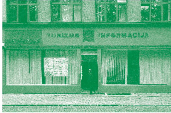
Laisvės Av. 36, the future Kaunas 2022 office, pre-renovation. 2018
