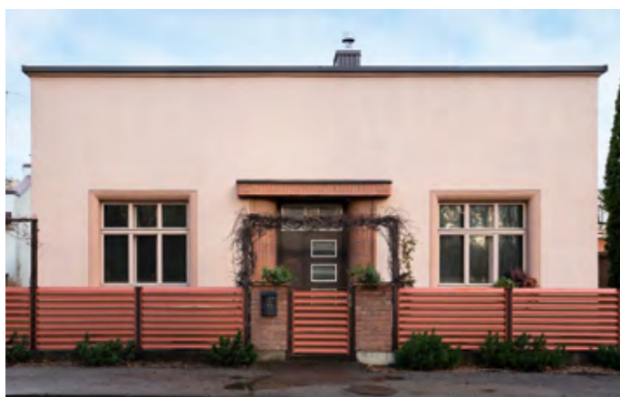
313. The front facade. Photo: Martynas Plepys, 2020
