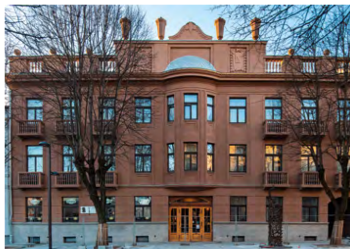
80. The Hotel Lietuva. The front facade. Photo: Martynas Plepys, 2020
