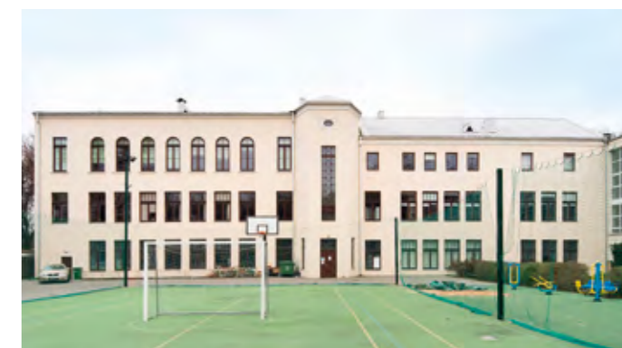
250. The rear facade. Photo: Martynas Plepys, 2020
