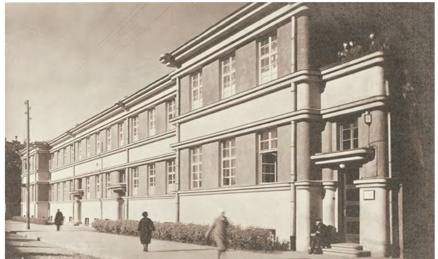
259. A new ENT Hospital hospital on 49 Vytauto Prospektas, designed by architect Vytautas Landsbergis in 1928. Photo: Private collection
