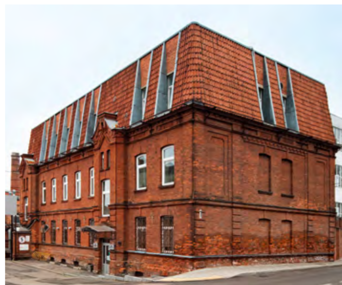
267. Administrative building. Photo: Martynas Plepys, 2020
