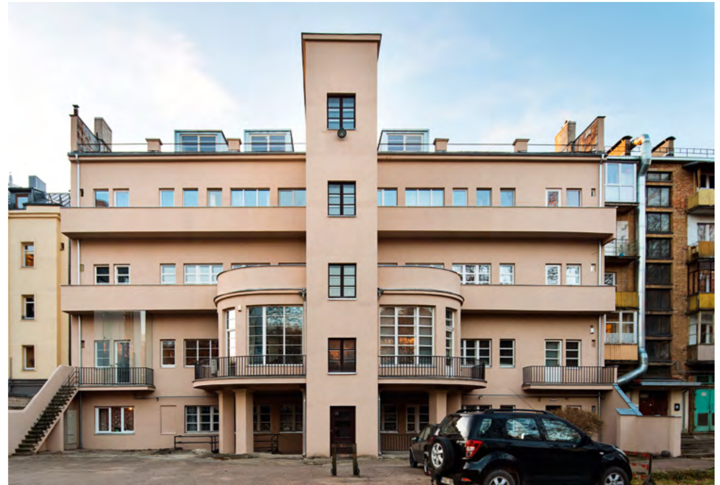
181. The rear facade. Photo: Martynas Plepys, 2020
