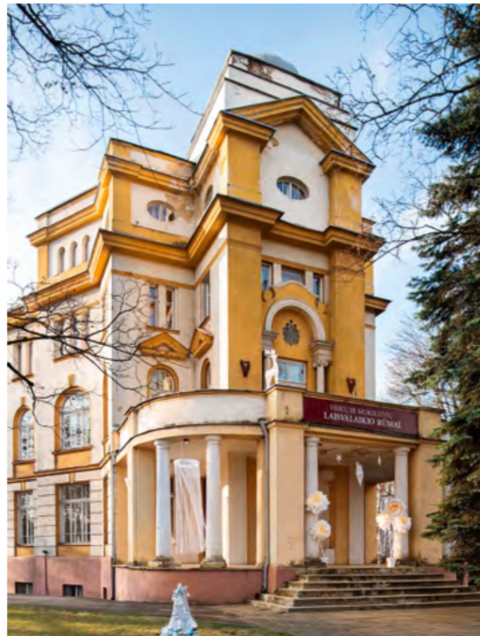
358. The main facade. Photo: Martynas Plepys, 2020
