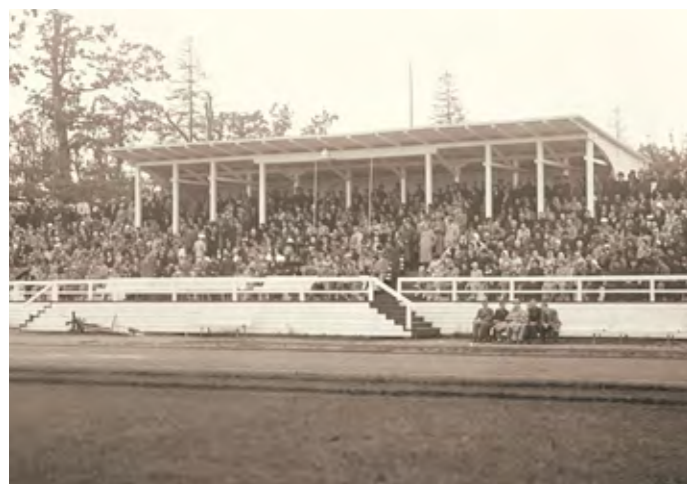
403. The Kaunas Stadium in the 1930s. Photo: LCVA
