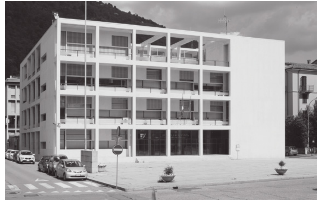
Figure 1. Giuseppe Terragni, Casa del Fascio (Fascist Party headquarters), Como 1936. Photograph Camilla Borghese.
