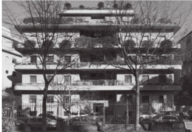
Figure 9. Camilla Borghese, Dialoghi Urbani (detail: Palazzina via Bruxelles 47, Rome, Italy). Courtesy Camilla Borghese.
