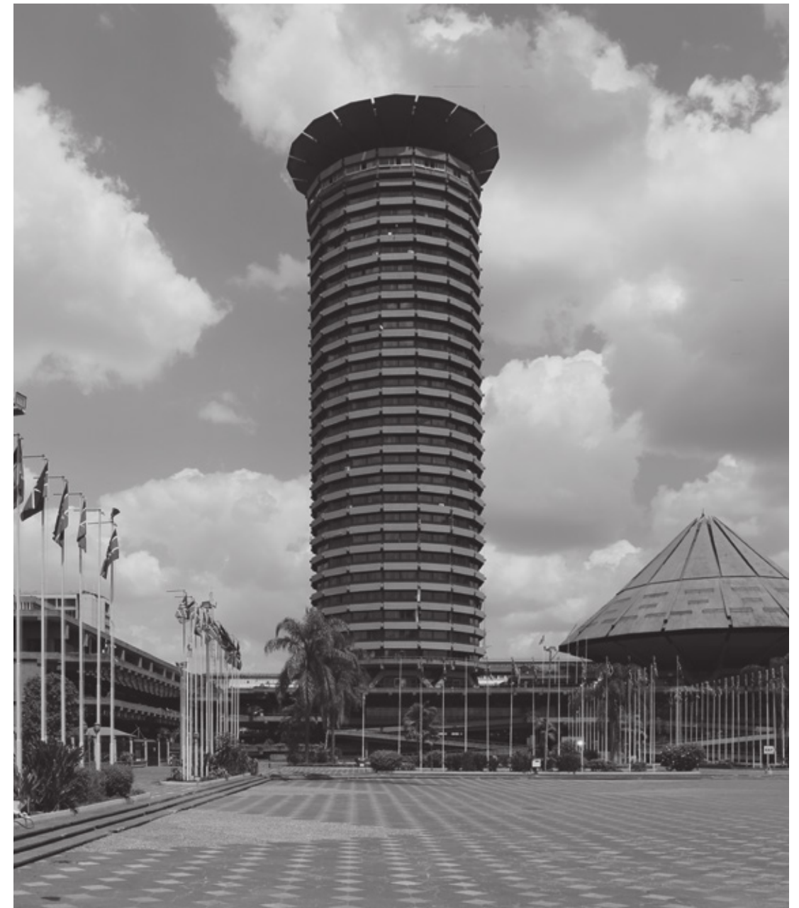
Figure 5. The 105-metre-high Kenyatta International Convention Centre in Nairobi (1973), designed by David Mutiso and Karl Henrik Nøstvik, which became a powerful architectural symbol of Kenyan independence and an icon of a burgeoning capital. Photograph Edward Denison
