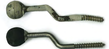
Originalus, restauruotas lango „muštukas“ (stabdis) Original restored window stopper
